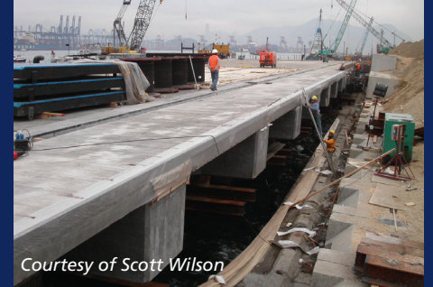
Container Terminal No. 9, Hong Kong
