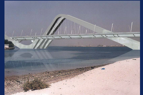
Sheikh Zayed bridge, Abu Dhabi, UAE
