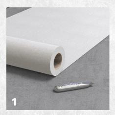
FA Impact 21 is laid on top of the concrete floor, which must be free of dust.
