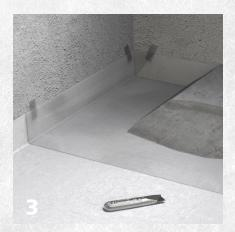
For walls, FA Impact 21 and the plastic foil are pulled up lengthwise of the wall. Corners are cut using a Stanley knife and secured with tape. Concrete can then be cast according to the instructions from the supplier.
