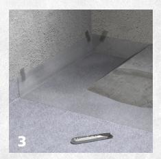
For walls, FA Impact 19 and the plastic foil are pulled up lengthwise of the wall. Corners are cut using a Stanley knife and secured with tape. Concrete can then be cast according to the instructions from the supplier.
