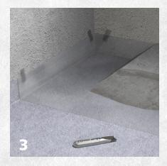
For walls, FA Impact 18 and the plastic foil are pulled up lengthwise of the wall. Corners are cut using a Stanley knife and secured with tape. Concrete can then be cast according to the instructions from the supplier.
