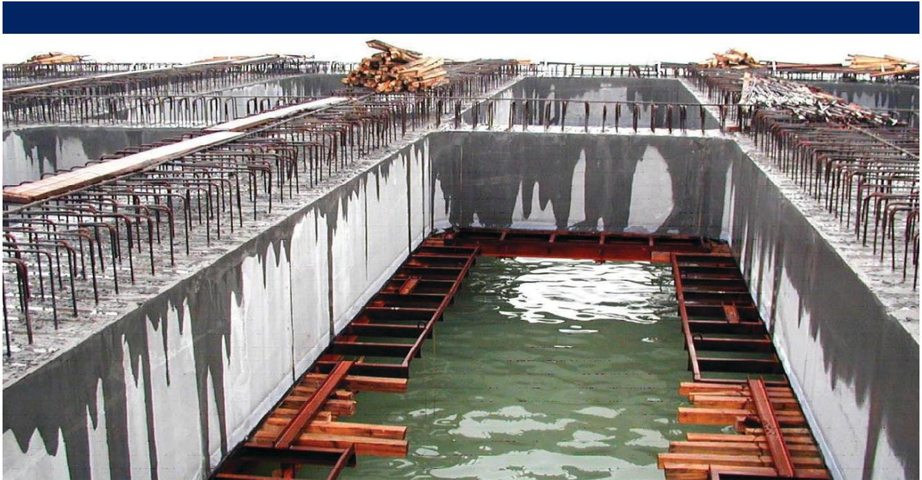
When the construction of the quay for Shekou Container terminal was commenced in December 2002, Controlled Permeability Formwork was not specified. However, the client wanted a dense concrete surface to protect the quays from the constant exposure to salt water, and thereby achieve a longer service life with reduced maintenance costs. Formtex® CPF liner was then chosen to secure a dense concrete with extended durability in this aggressive environment.
