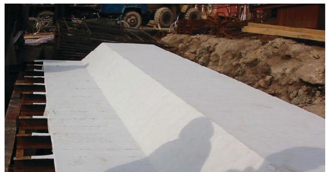
Figure 3. Casting of parapet and finished result.
