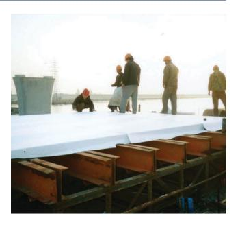
No form size is too small or too big to use Formtex® and this case's forms were as big as  $4 \times 12 \text{ m}$ . Bends or curves are no problems as Formtex® is a flexible material which will follow the contour of the form as seen on picture to the left with vertical installation.
