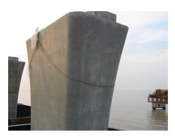
Finished piers, on their way to installation, with a smooth and dense concrete surface due to the usage of CPF Formtex®.
