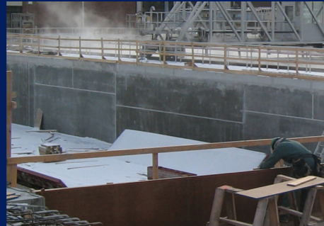
Waste water treatment plant, Canada
