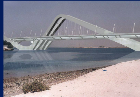
Most Sheikh Zayed, Abu Dhabi, UAE
