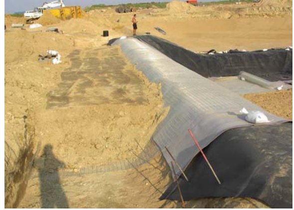
Figure 2: Anchorage of geogrid in anchor trench
