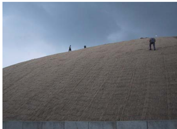
Figure 7: Installation of erosion control mat
