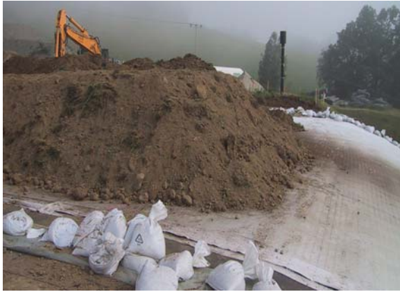
Figure 1: Anchorage of geogrid in runout area
