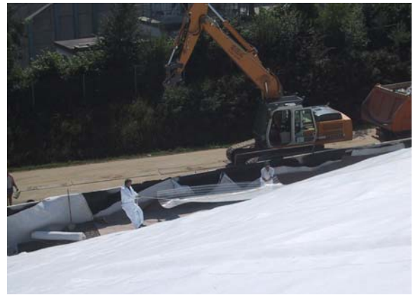
Figure 4: Pulling geogrid tight
