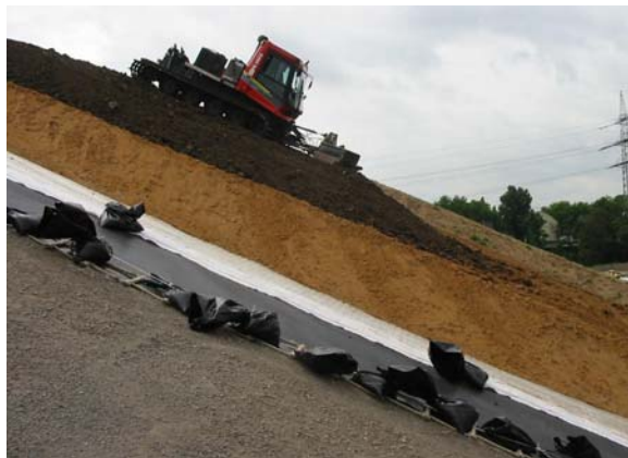
Figure 5: Installation of cover from top to bottom using lightweight dozer
