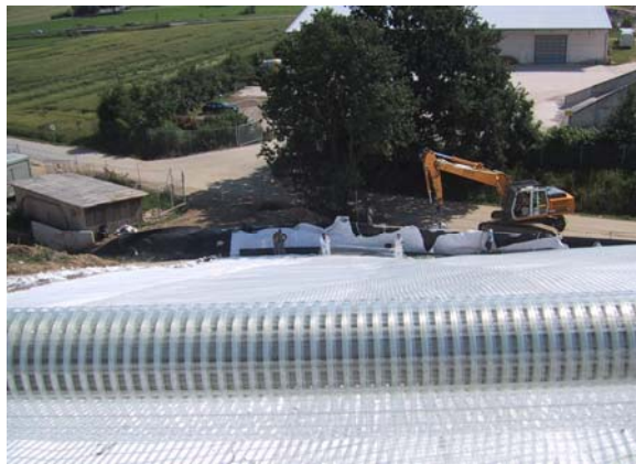
Figure 3: Unrolling geogrid from top to bottom
