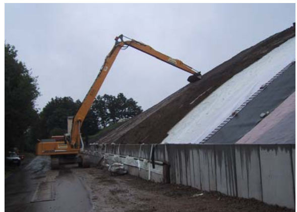
Figure 6: Installation of cover soil with long-boom excavator
