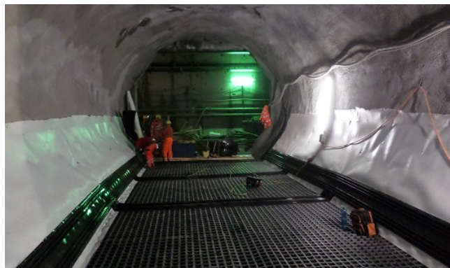
Fig 5: Cavidrain Invert installed ready for concrete infill
