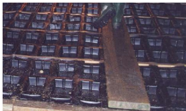
Fig. 3: Use spreader boards during installation
