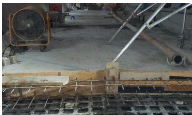
Fig 6: Formwork placed along rib of Cavidrain Invert
