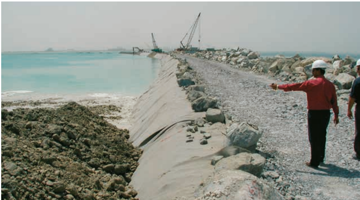
Source: Palm Island, Dubai. Installation of Fibertex F-650M. The Fibertex Geotextile will be covered completely with gravel and sand.
