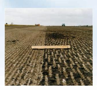
Fibertex AM-2 functions as a stress-absorbing membrane which prevents cracks in the existing road surface from reflecting up through the new asphalt wearing course.
