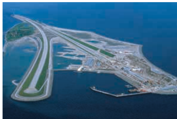
Figure 1.3: Le Great Belt traversant le Danemark
