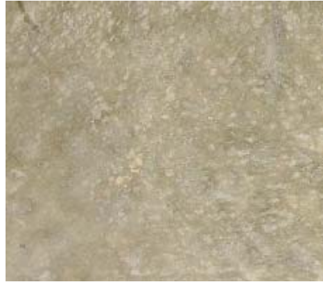
Fig. 14 Concrete cast using Formtex CPF
