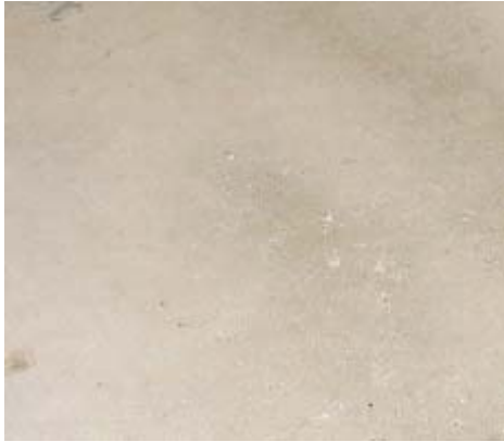
Fig. 13 Concrete cast using IF
