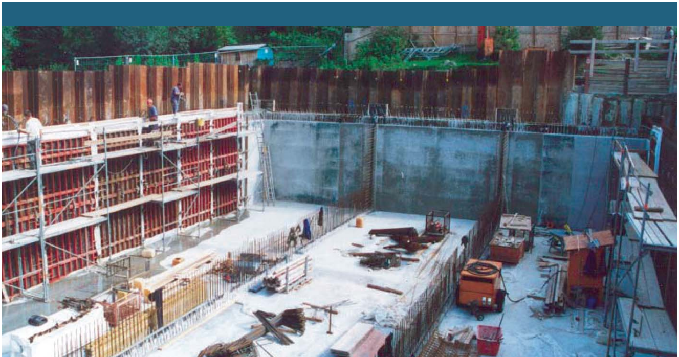
Figure 1. The casting of the west wall.
