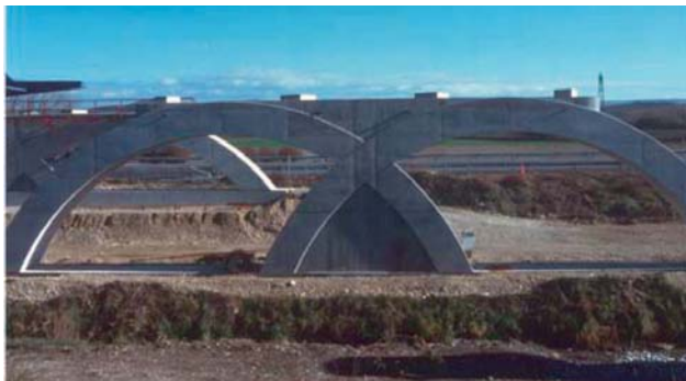
Figure 2. Bridge parapet cast with Formtex®.
