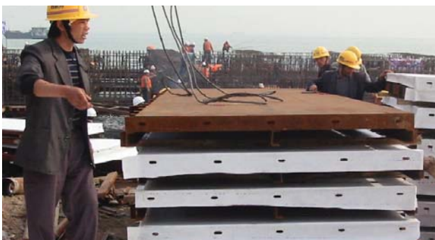
Figure 2. A formwork element lined with Formtex ® ready for casting.
