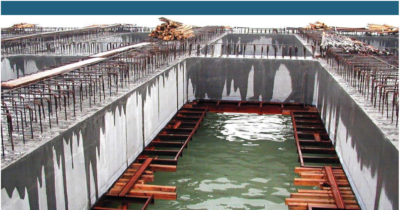
Figure 1. The construction site at Shekou Container Terminals.
