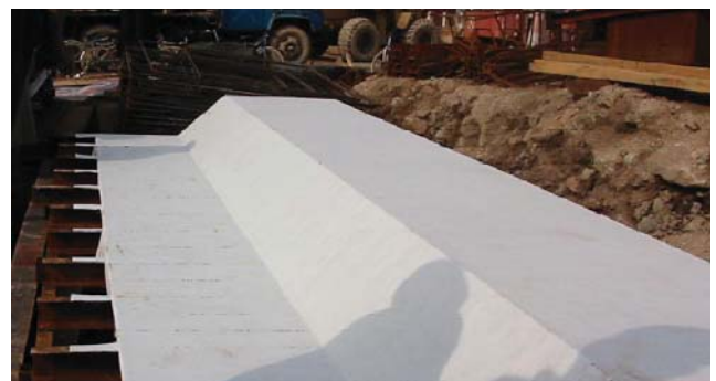
Figure 3. Casting of parapet and finished result.
