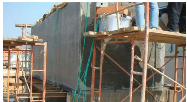
Figure 3. Concrete core sample is drilled for testing.
