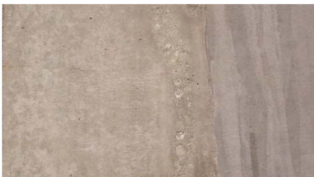
Figure 2. Concrete surface achieved without formliner (left) and with Formtex® (right).
