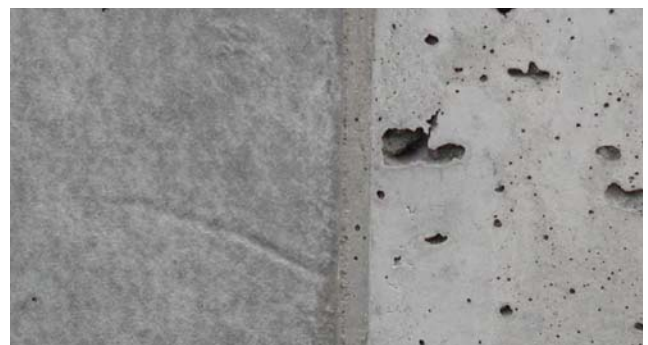
Figure 3. Concrete surface achieved with Formtex® (left) and without Formtex® (right).
