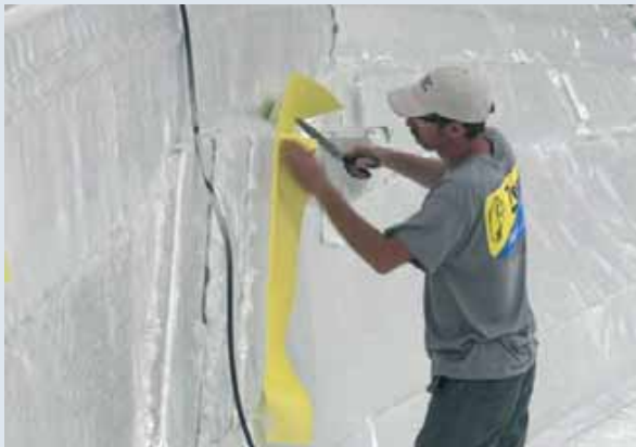
3. Compoflex® RF 3 is easy to cut using normal scissors.
