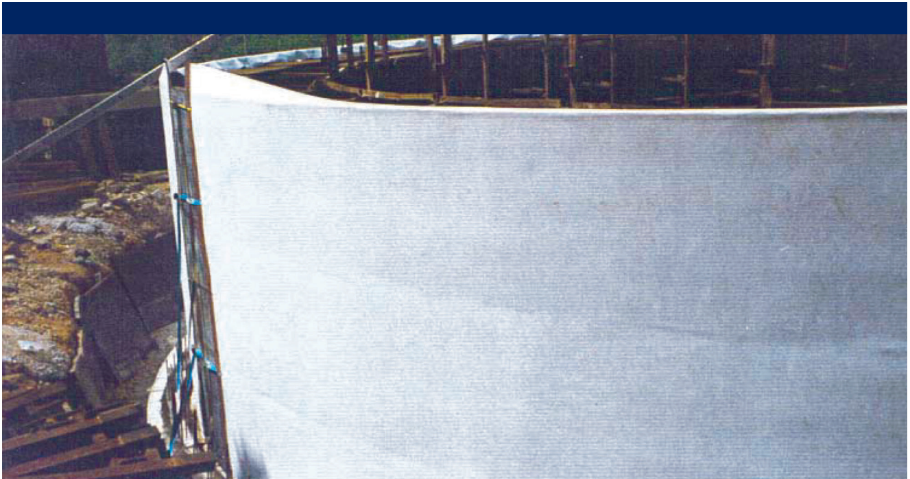
Figure 1. The formwork lined with Formtex® before casting of a wastewater tank for the sewage work.
