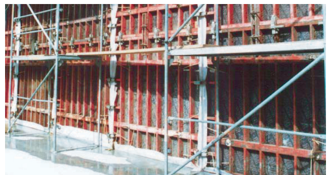
Figure 3. The concrete is vibrated and the water escapes under the formwork.
