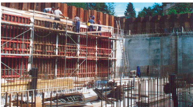
Figure 2. Casting of the west wall.
