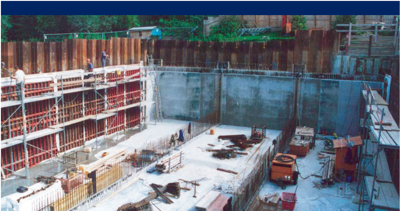
Figure 1. The casting of the west wall.
