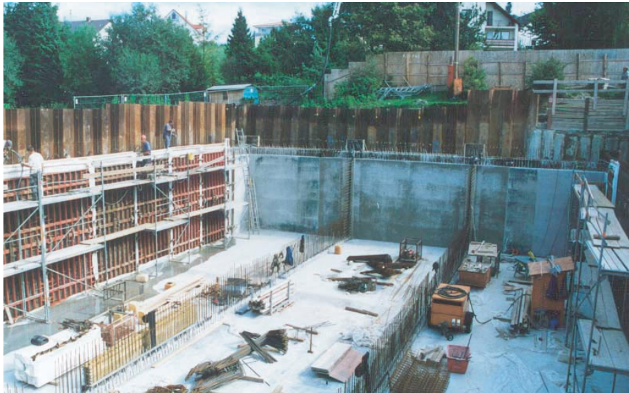
The casting of the west-wall and the finished north-wall
