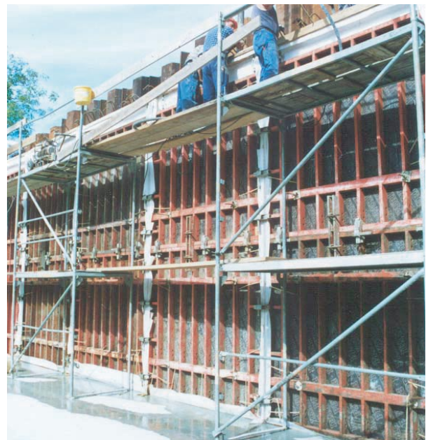
The concrete is vibrated and the water escapes under the formwork
