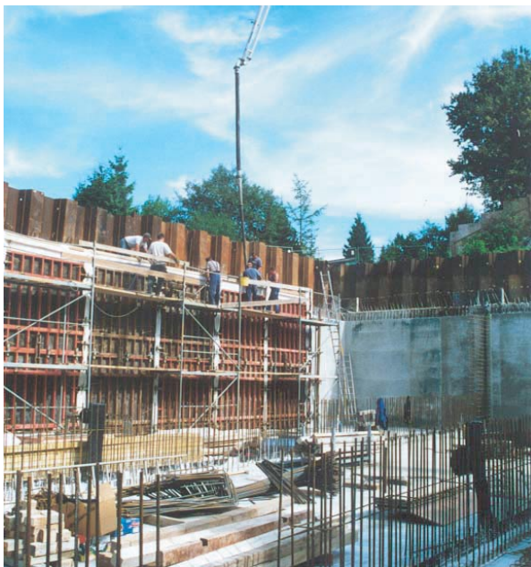
Casting of the west-wall
