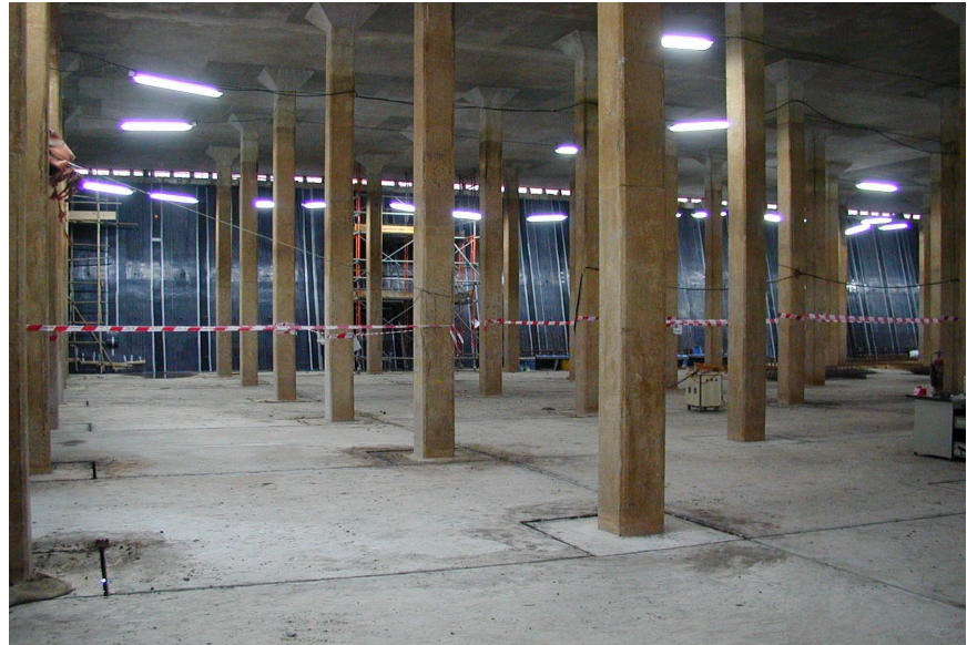
Figure 1: The construction site of Water Service Reservoir
