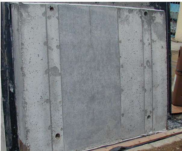
Figure 2. A trial for installation of Formtex ® (middle)
