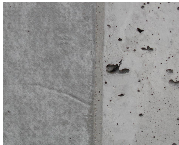
Figure 3. Concrete surface achieved with Formtex ® (Left) and without Formtex ® (Right)
