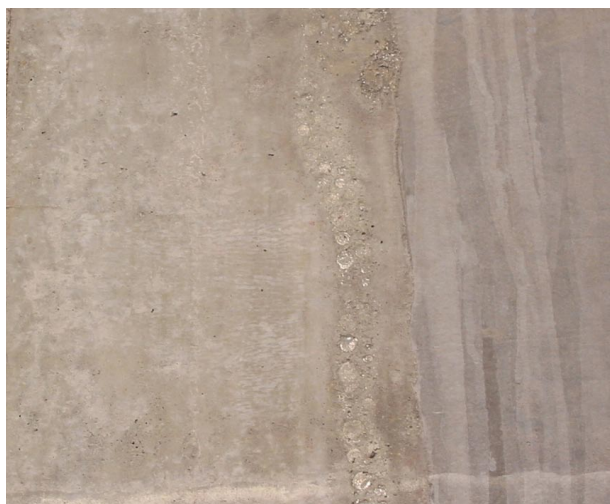
Figure 2. Concrete surface achieved without formliner (left) and with Formtex ® (right)
