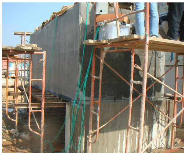
Figure 3. Concrete core sample is drilled for testing.
