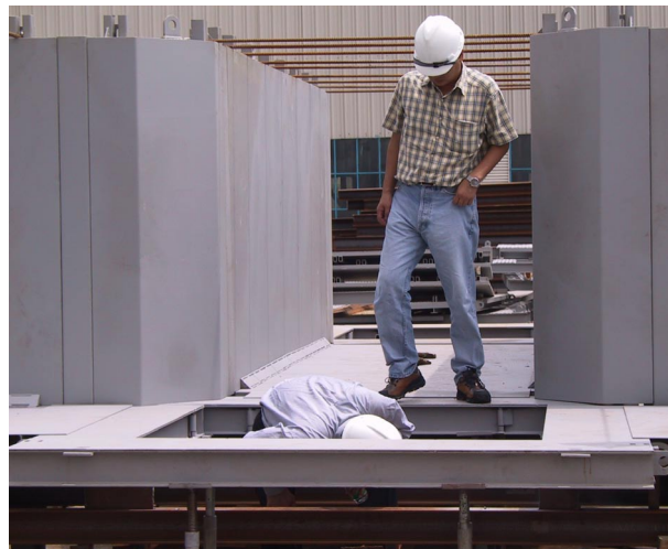
Figure 5. The formwork for the huge beams is inspected.
