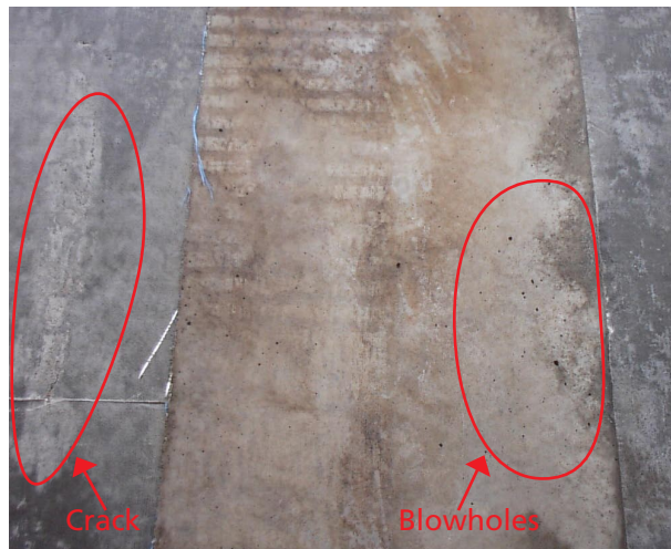
Figure 3. Achieved concrete for competing product (Left), without formliner (middle) and Formtex ® (right)
