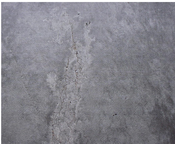
Figure 6. A large crack in the surface of the test of the competing product.
