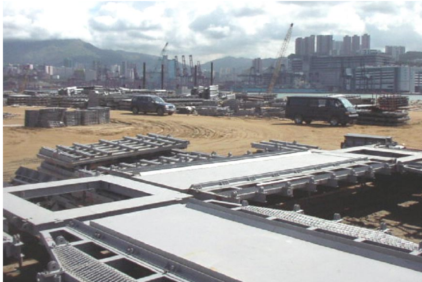
Figure 1. The construction site at Container terminal No. 9.
