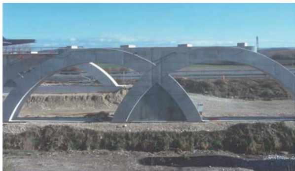
Bridge parapet cast with Formtex ® .
