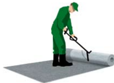
Fig 5. When unrolling Fibertex AM2 manually, using a pushing tool makes it easier to keep the direction and avoid wrinkles.
