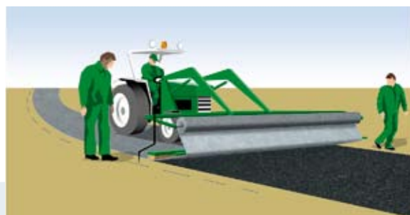
Fig. 6. Mechanical unrolling of Fibertex AM2 Special is fast and minimises wrinkles even in soft curves.
