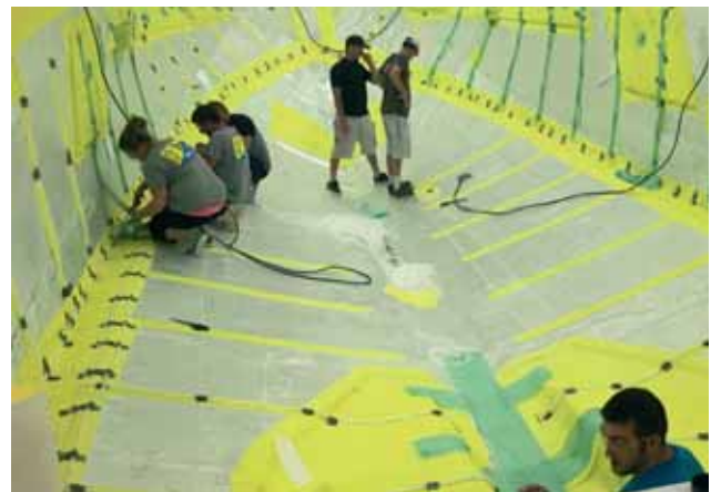
4. For easy removal and quick infusion, feed lines are mounted directly on Compoflex® RF 3. There are 17 feed points, 8 on the hull bottom, 8 on the topsides and one on CL.
