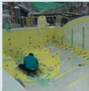
Overlapping is no problem with Compoflex® RF 3 due to the microporous surface.
